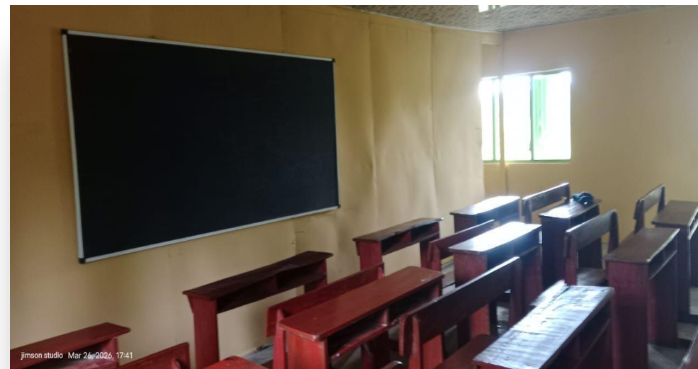
Ajide (Classroom) Renovation
