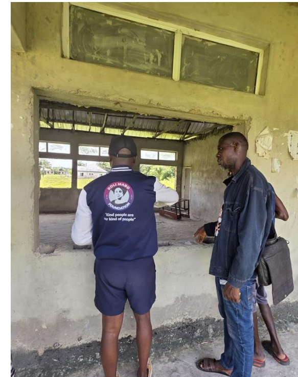
Roli Mabo Team, checking the renovation progress of Ajide Primary School
